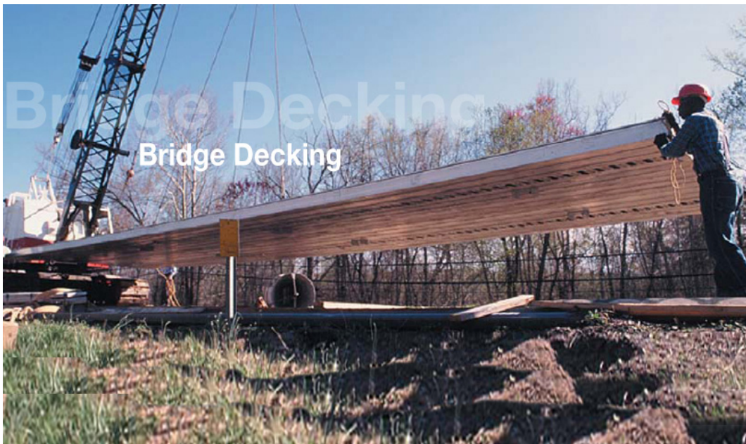
Figure 1: Sapa bridge deck
